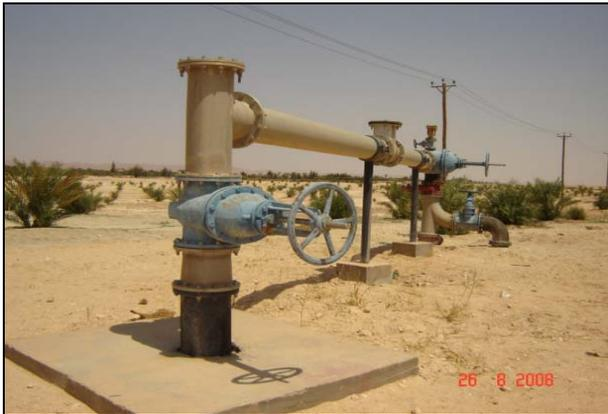
Fig. 1 Artesian well heat source.
