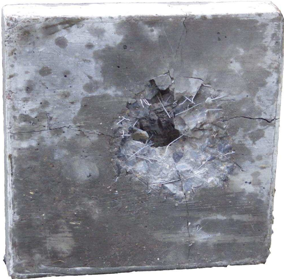
Figure 11 – Rear face of steel fibre slab
