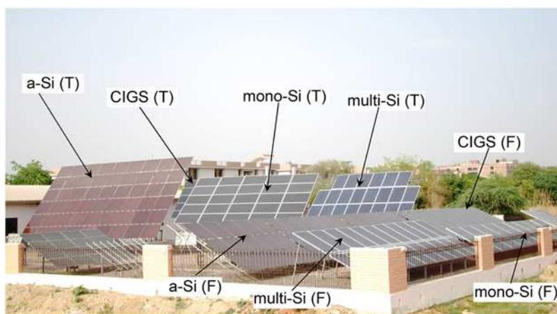
Fig. 1 PV systems installed at SERE
