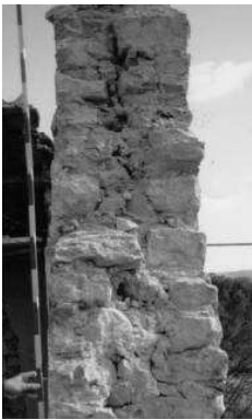
Figure 1 Double leaf wall
